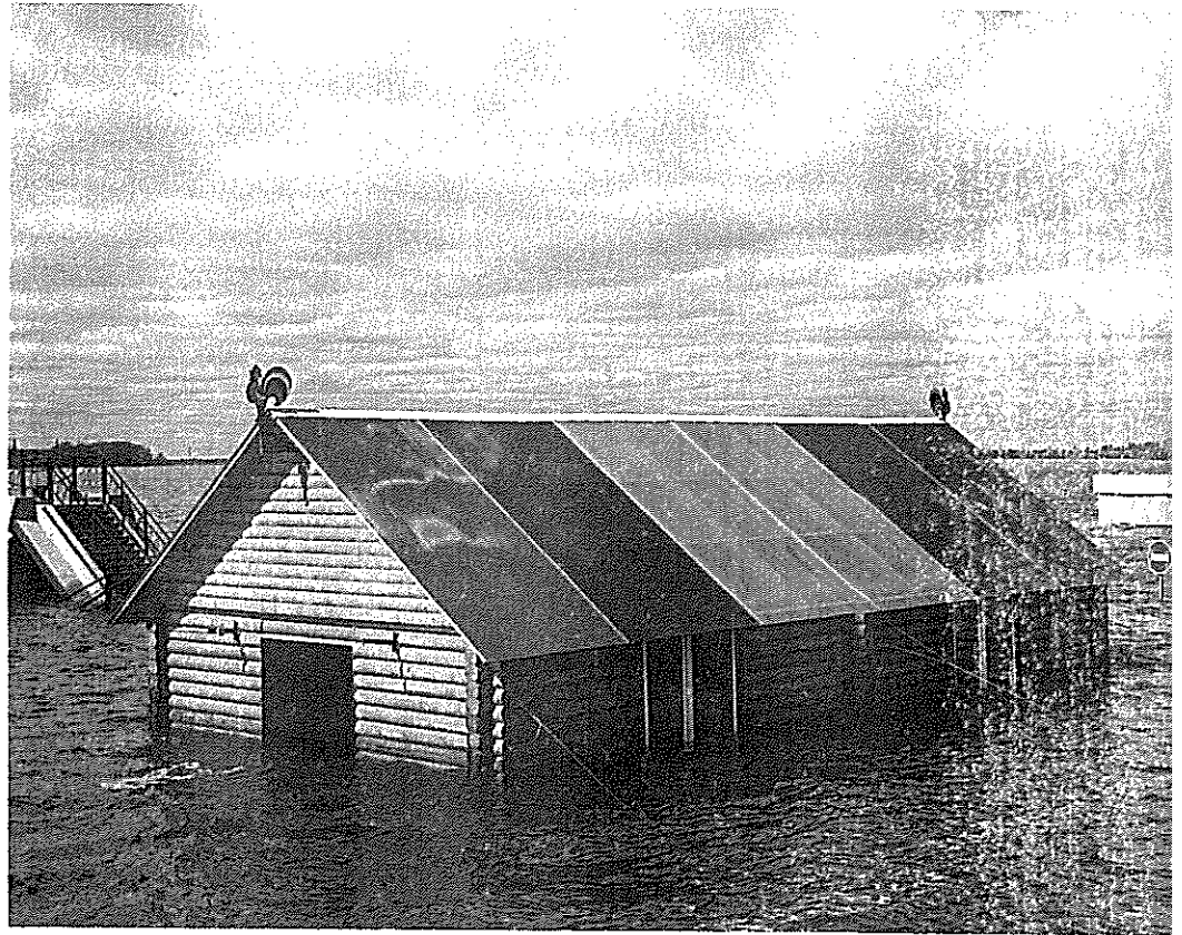
▲ Floodwaters damage homes and cars.
